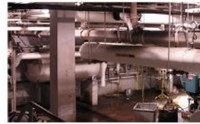
Draining water from the basement
